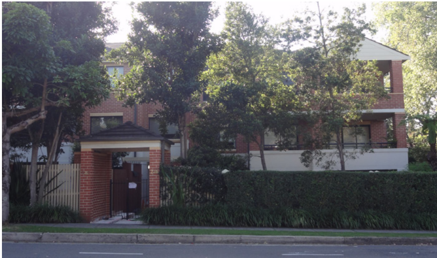
Existing 3 storey residential building further to the north
