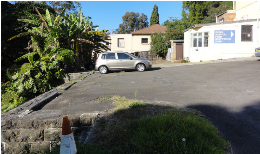
Rear surface car parking and retaining wall
