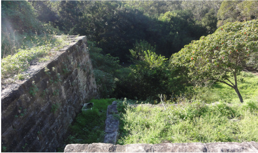
Steep slope with retaining wall to the south-eastern corner of the site
