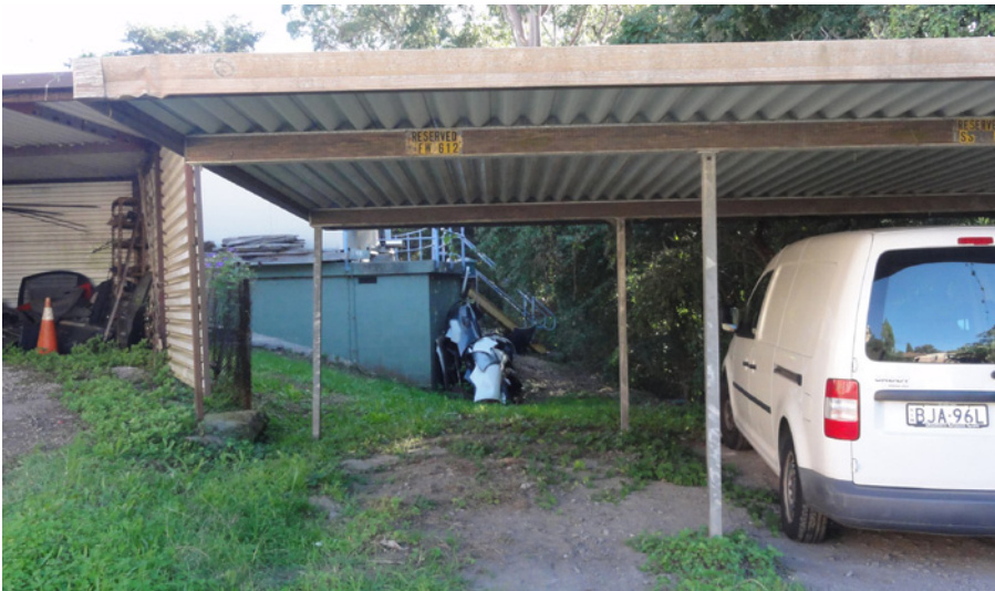
Existing structure and change of level at the rear boundary of the site
